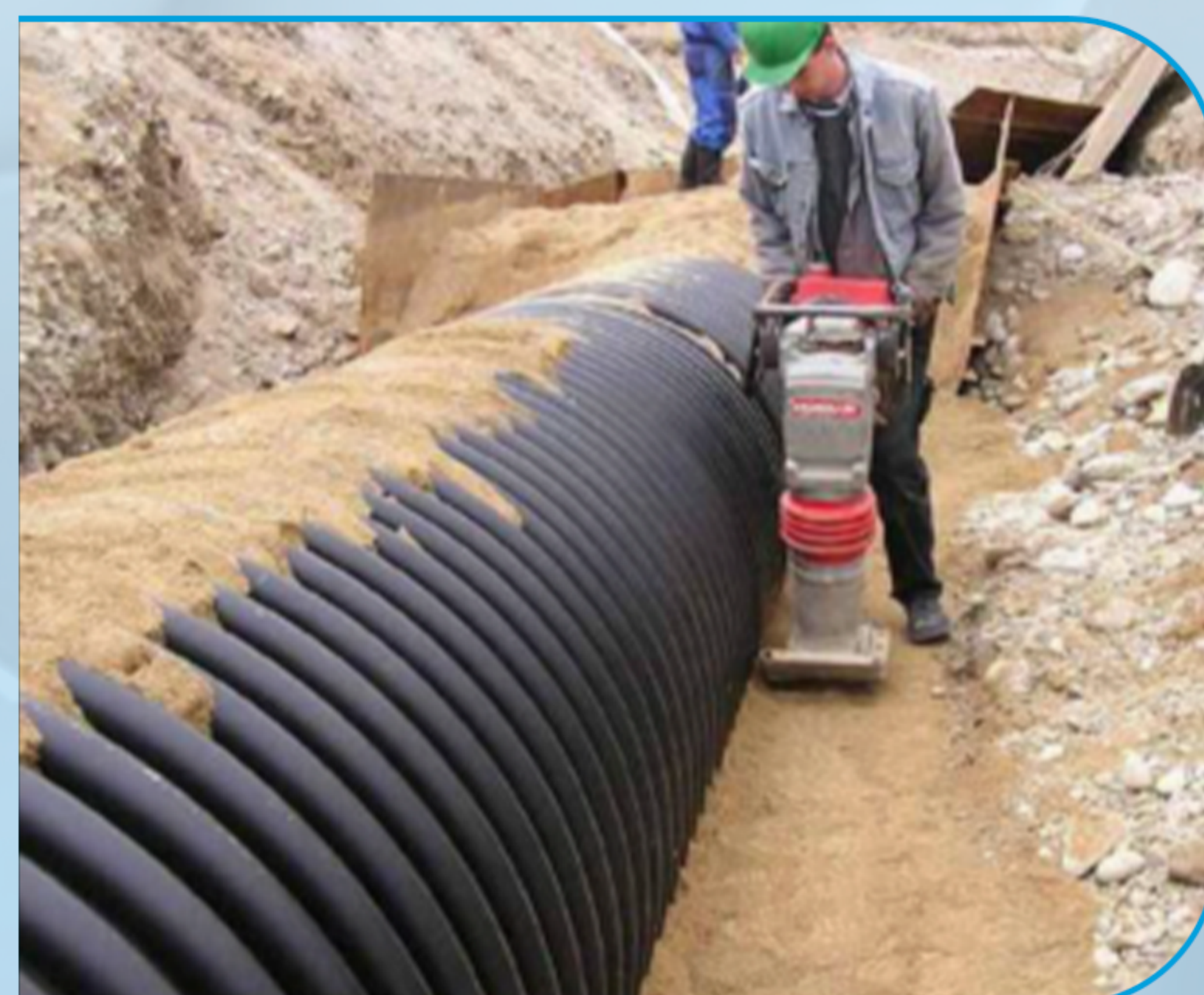
Compaction work with a vibratory plate
