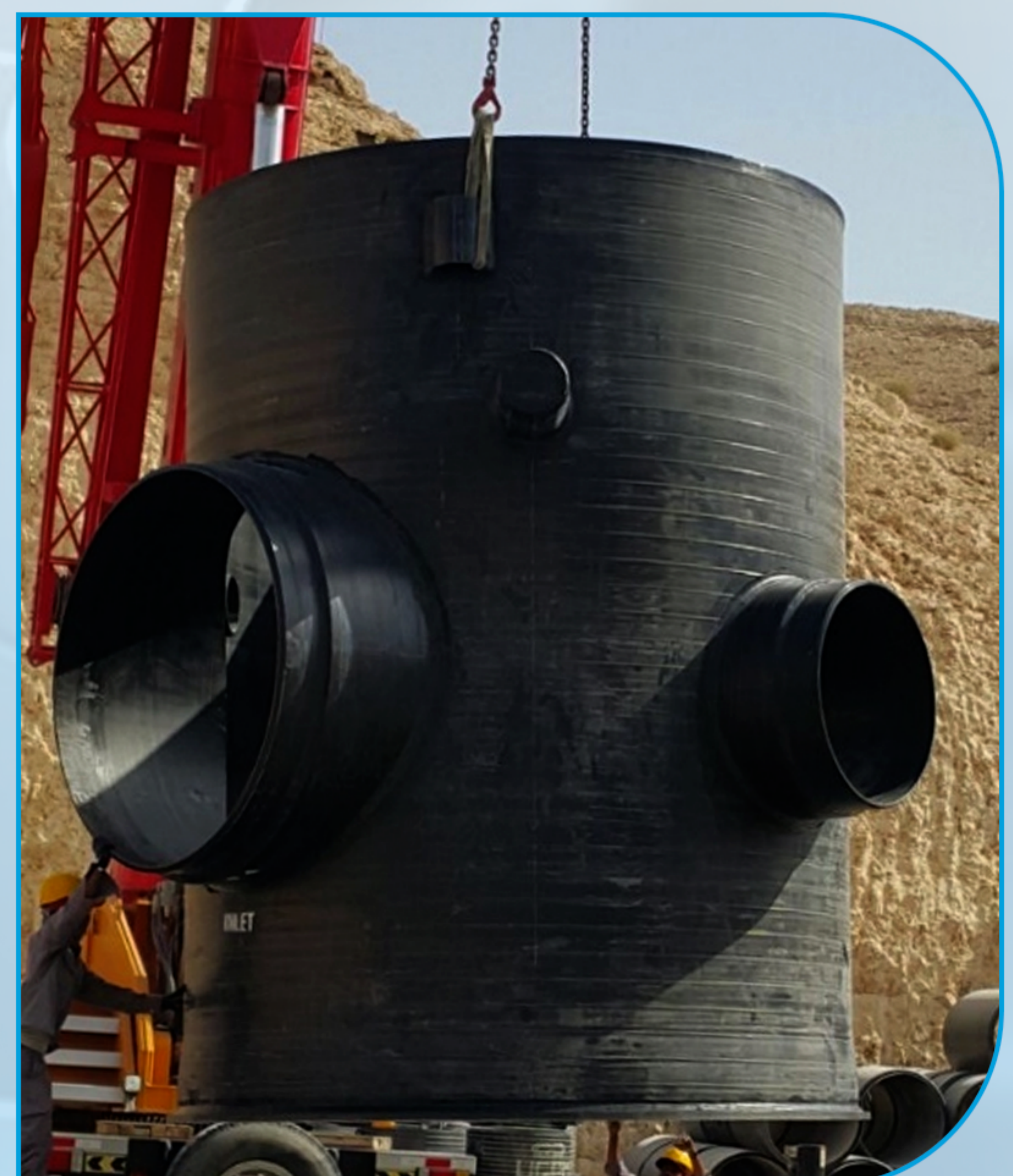
Unloading of Manholes
