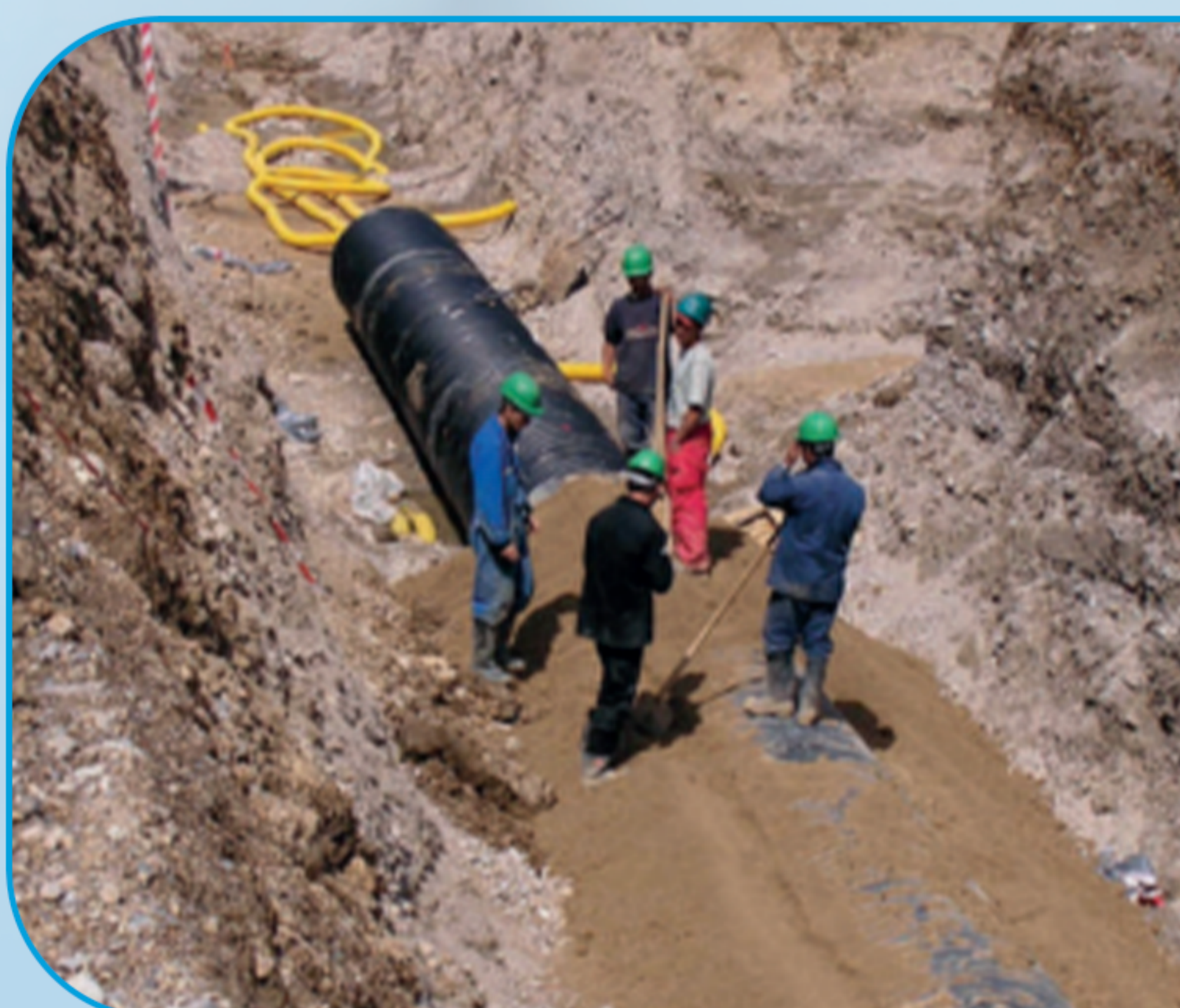
Compaction of main backfilling
